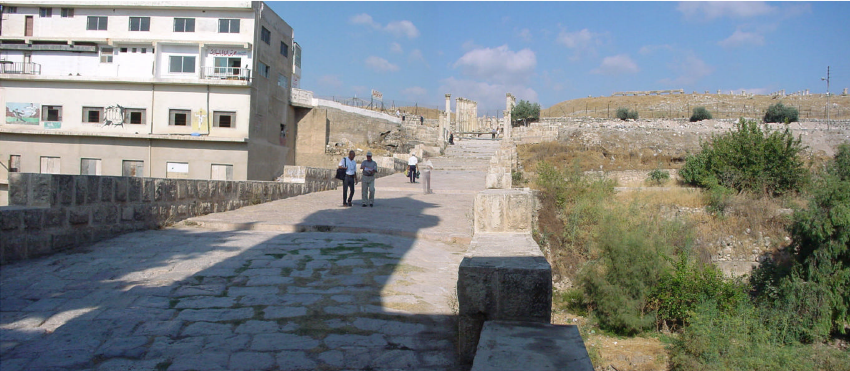
VIEWS OF THE WADI FROM THE SOUTH BRIDGE (ON THE LEFT: INTRUSIVE PRIVATE BUILDING)
