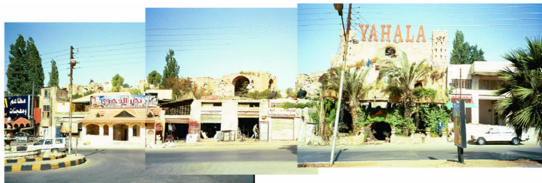
VIEW OF THE PRIVATE BUILDINGS WHICH NEED FAÇADE REHABILITATION
